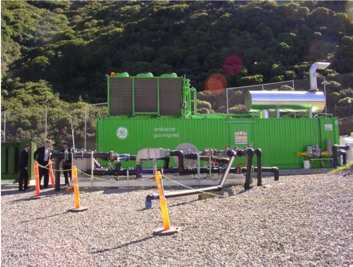
Todd Energy's LFG Generator on Wellington Landfill 2008
