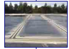
Weight pipes in position on a pond cover:
