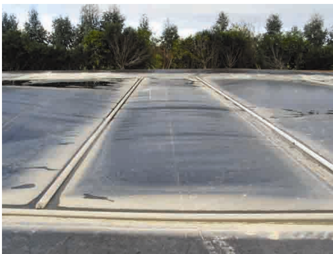
Weight pipes in position on a pond cover:
