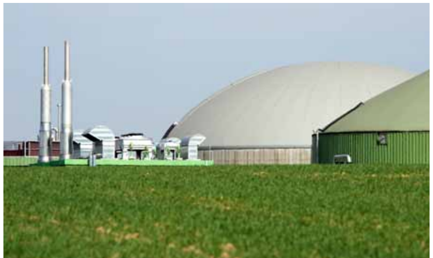
Biogas energy plant in Germany. Biogas already provides more than 3% of the whole of Germany's electricity consumption, as well as significant amounts of industrial heat, transport fuels, and volume injected into the natural gas grid.
