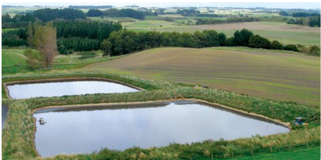
Ponds used for effluent disposal can provide the raw material for a biogas system. Covers also help to reduce odour.
