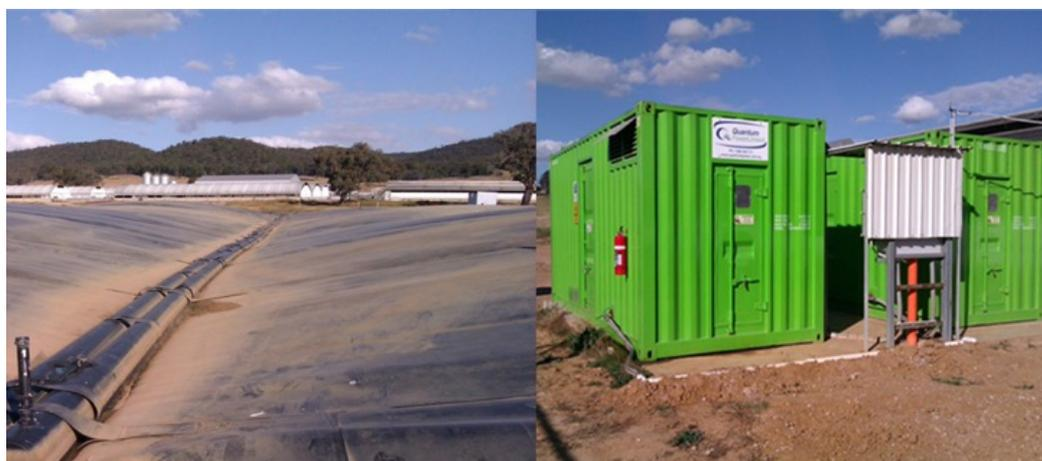
**Figure 7-1: High Density Polyethylene (HDPE) covered anaerobic lagoon (left) and combined heat and power (CHP) unit (right)**
