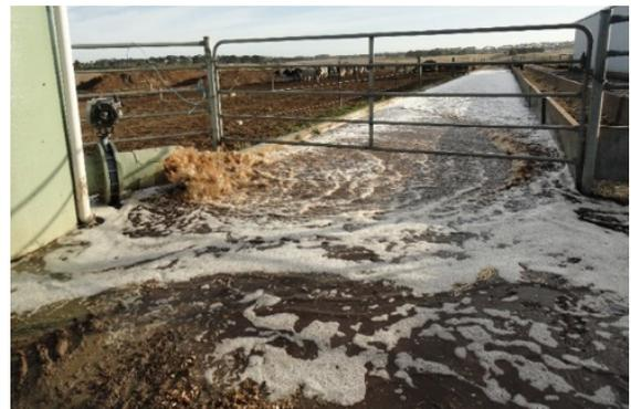
**Figure 3-1: Typical dairy effluent systems used on-farm in Australia, showing a flush tank being used for flushing of a dairy feed pad area.**
